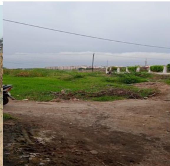
PANDIAN SALAI LIFT STATION – LS02
