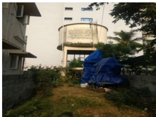
VGP AVENUE LIFT STATION – LS03
