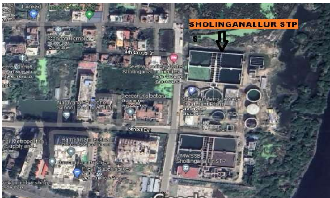
Figure 7: Location of existing Sewage Treatment Plant at Sholinganallur
