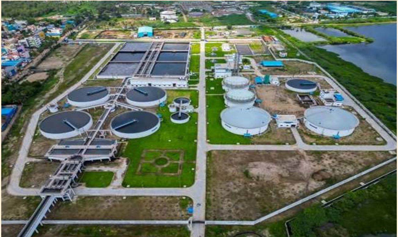
120 MLD (Zone – 2) Sewage treatment plant at Kodungaiyur.
