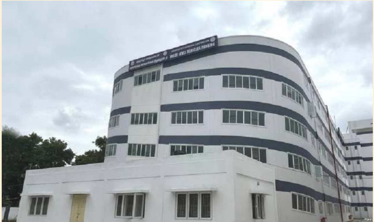
Construction of Multi Level Car Parking in Tiruppur Corporation Scheme: Smart City Mission, Project Cost: Rs. 12.87 Crore
