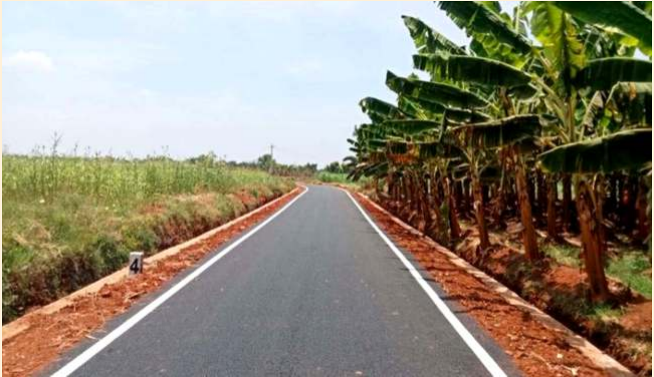
Construction of BT Road and Retaining wall at Valliyampalayam road, Vellankattupalayam in Lakkampatti Town Panchayat, Erode District. Estimate Cost: 1.22 Crore
