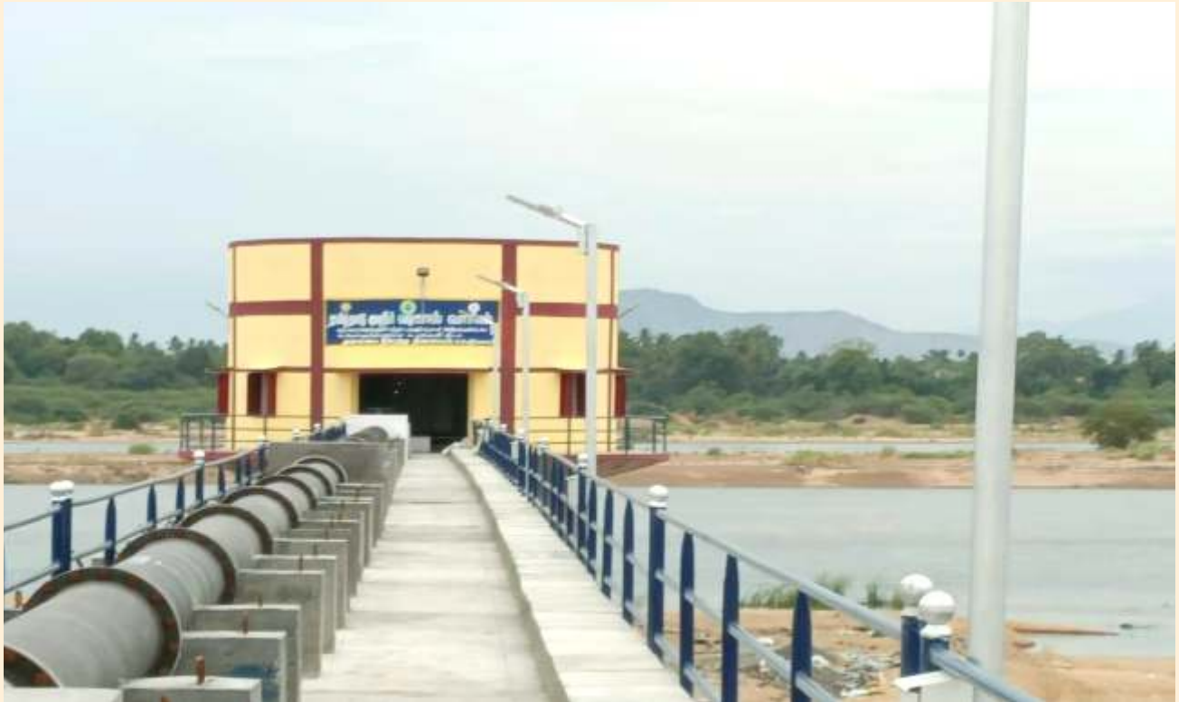
CWSS to 756 rural habitations in K.Paramathi and Aravakurichi unions in Karur district, Head works – Sevanthipalayam
