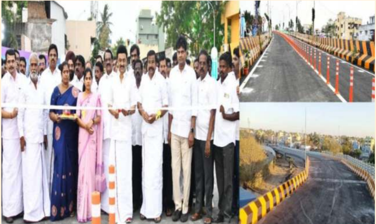
The Hon'ble Chief Minister of Tamil Nadu Thiru. M. K Stalin inaugurated the newly constructed Rail over Bridge (ROB) at the cost of Rs. 61.98 Crore connecting Kolathur with Villivakkam on 13.05.2023.
