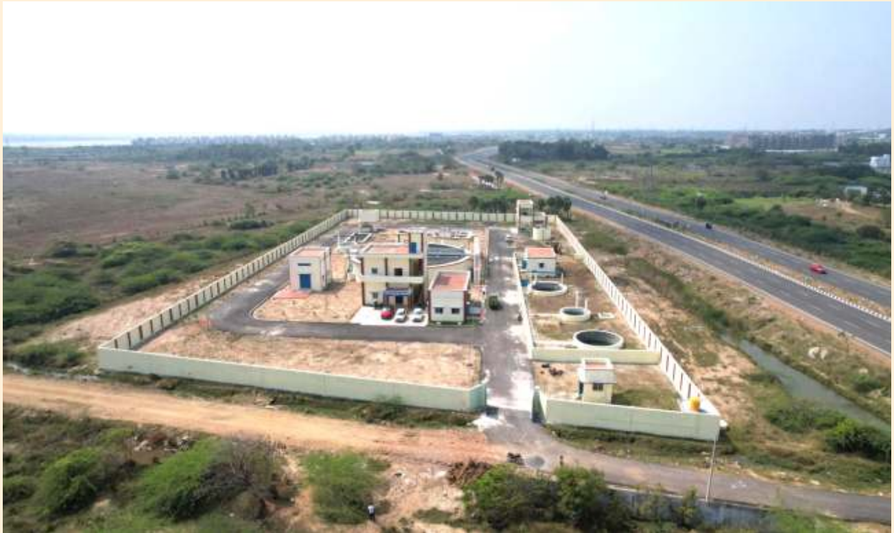
UGSS to Tiruporur Town Panchayat, Chengalpattu District. 4.02 MLD capacity Sewerage Treatment Plant at Kalavakkam.
