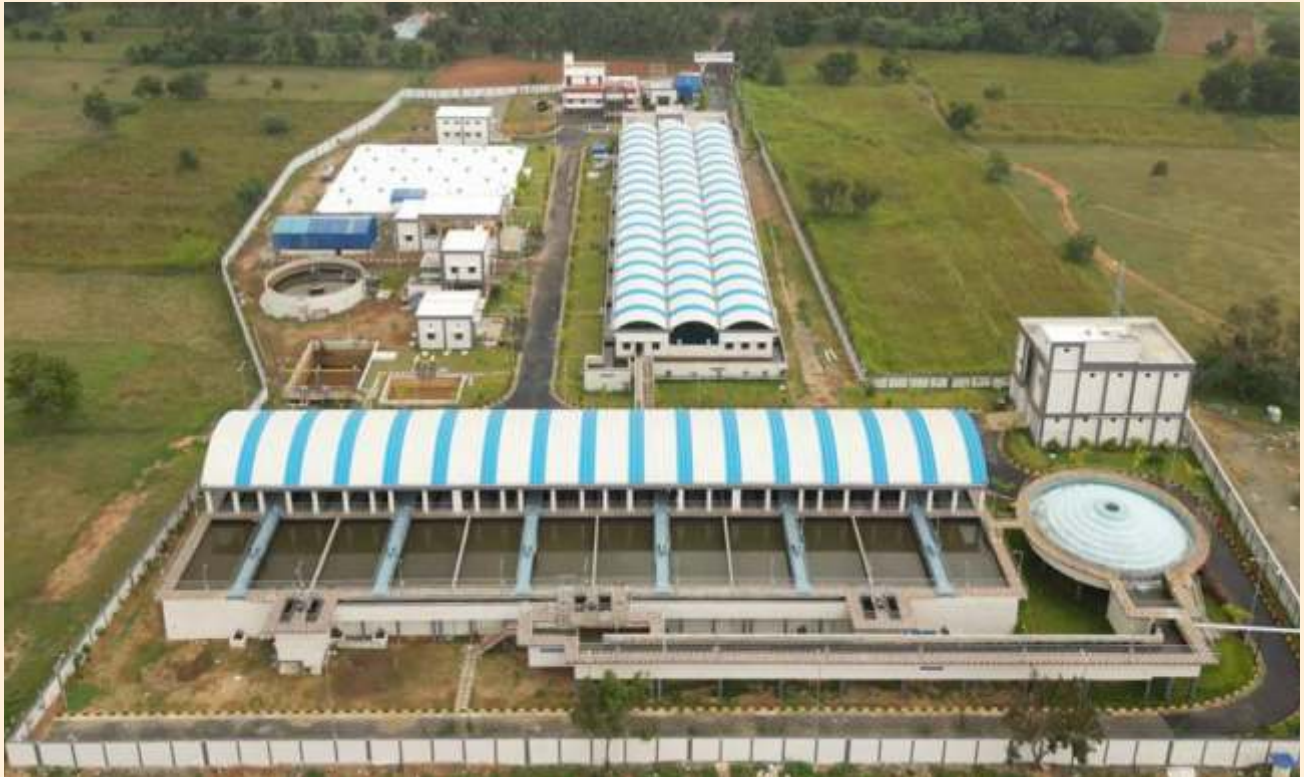
Construction of Water Treatment Plant in Tiruppur Corporation under AMRUT, Project Cost: Rs. 1120.57 crore
