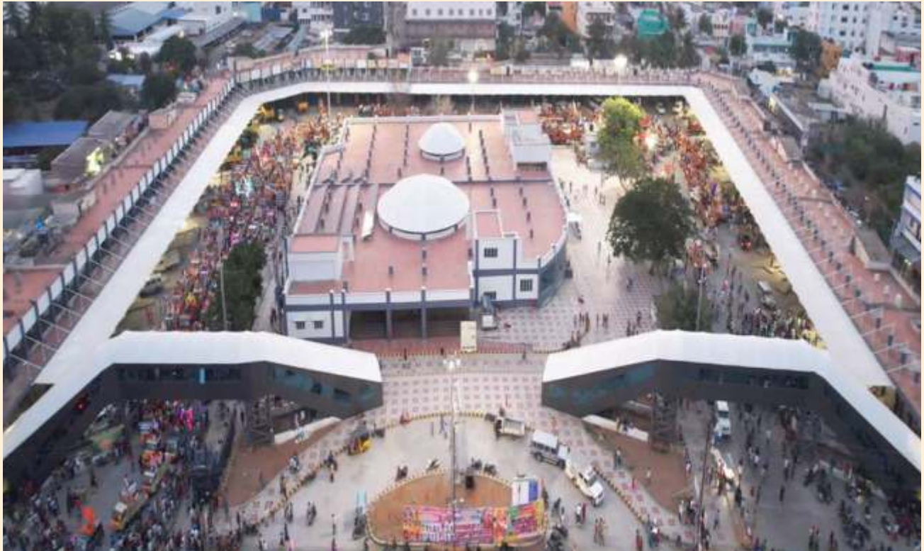
Redevelopment of Bus Stand in Tiruppur Corporation Scheme: Smart City Mission, Project Cost: Rs. 30.60 Crore
