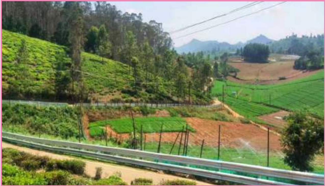
Provision of crash barrier along the road from Muttinadu to Kolanimmattam in Adigaratty town panchayat (The Nilgiris district),
