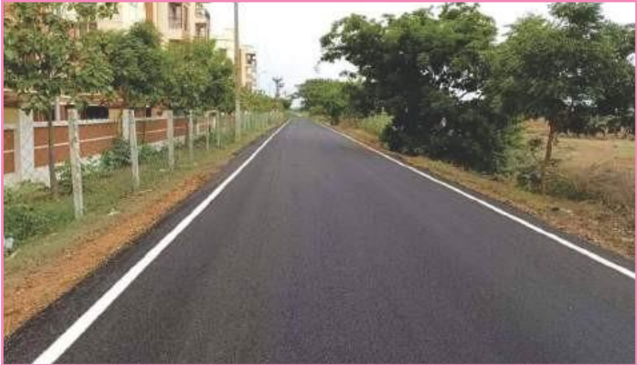
Construction of a new BT road (earthen road to BT road) in Thiruporur town panchayat (Chengalpattu district), Scheme : Capital Grant Fund; Project cost : Rs. 1.00 crore
