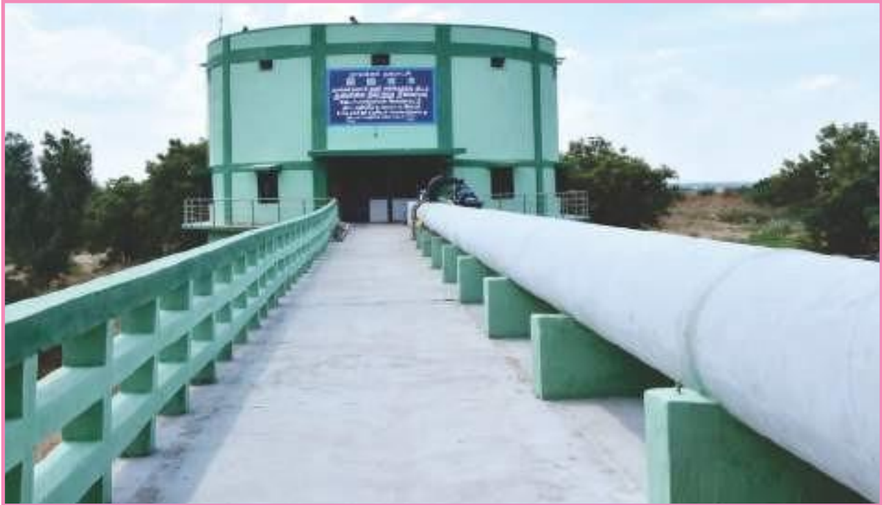
Head works at Jaderpalayam, Water supply improvement scheme to Namakkal municipality in Namakkal district
