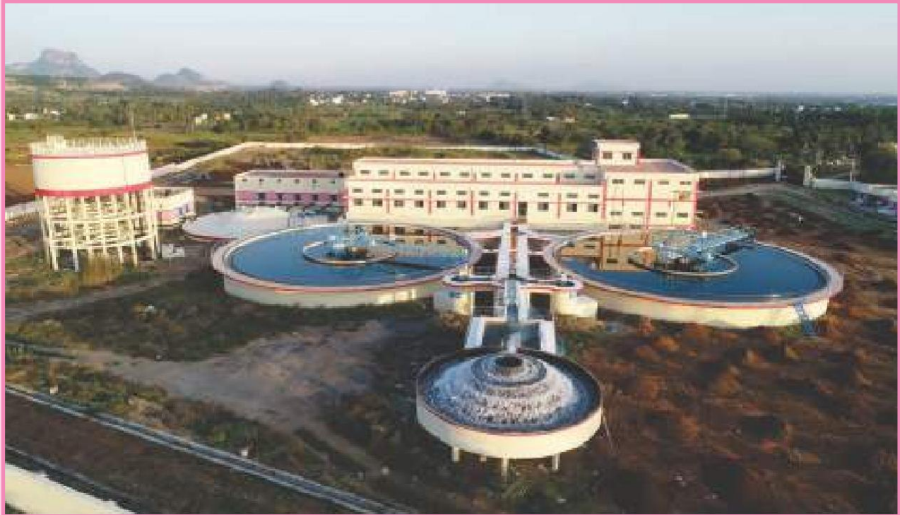
25.51 MLD capacity water treatment plant, constructed under CWSS to Sankari, Alampalayam and Padaveedu town panchayats and 669 rural habitations in Pallipalayam and Tiruchengode unions in Namakkal and Salem districts
