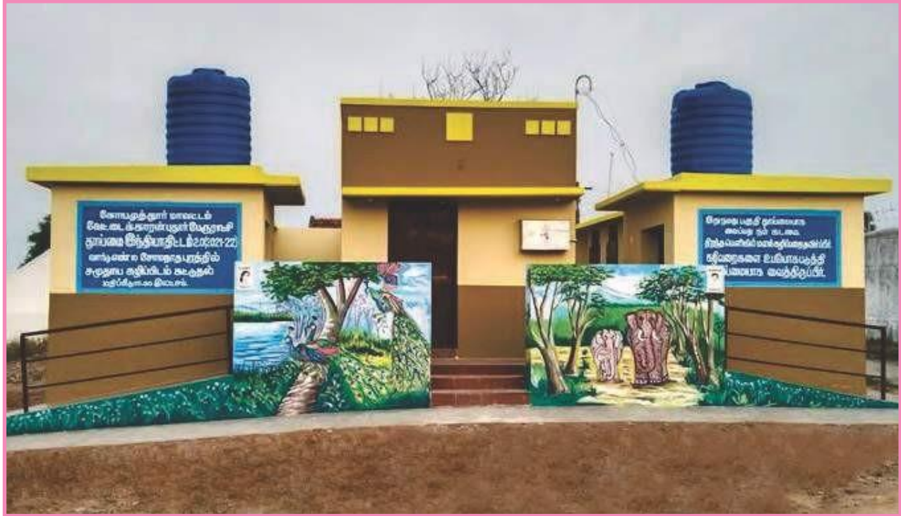
Construction of community toilet in Vettaikaran Pudhur town panchayat (Coimbatore district), Scheme : Swachh Bharath Mission 2.0; Project cost : Rs. 15.00 lakh
