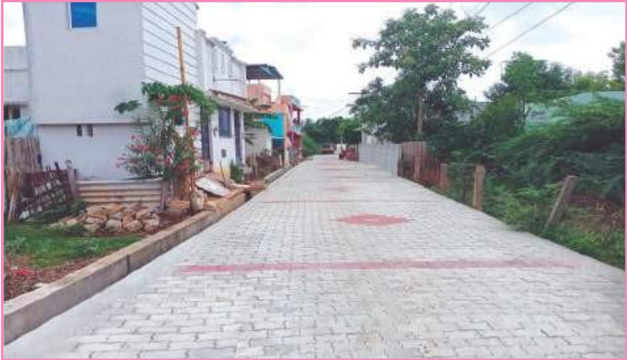
Construction of paver block pavement and stormwater drain in Thuvakudi municipality (Tiruchirapalli district), Scheme : Kalaignar Nagarapura Mempattu Thittam; Project cost : Rs. 28.70 lakh
