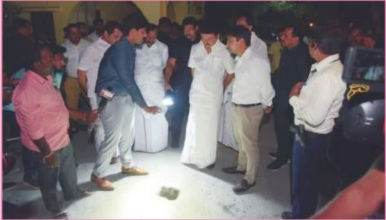
Honourable Chief Minister inspecting the quality of the road laid at PSG HUDCO colony at Peelamedu, Coimbatore Scheme : TURIP; Project cost : Rs. 1.28 crore
