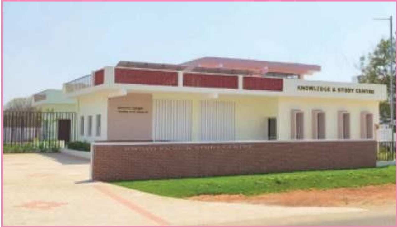
Construction of library cum knowledge centre building in Namakkal municipality, Scheme : Kalaingar Nagarpura Mempattu Thittam; Project cost : Rs. 2.00 crore
