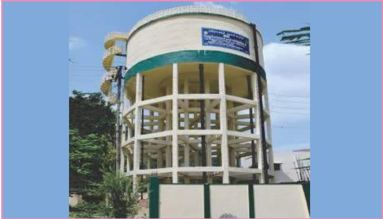
10 lakh litre capacity overhead tank constructed under water supply improvement scheme to Vellore corporation
