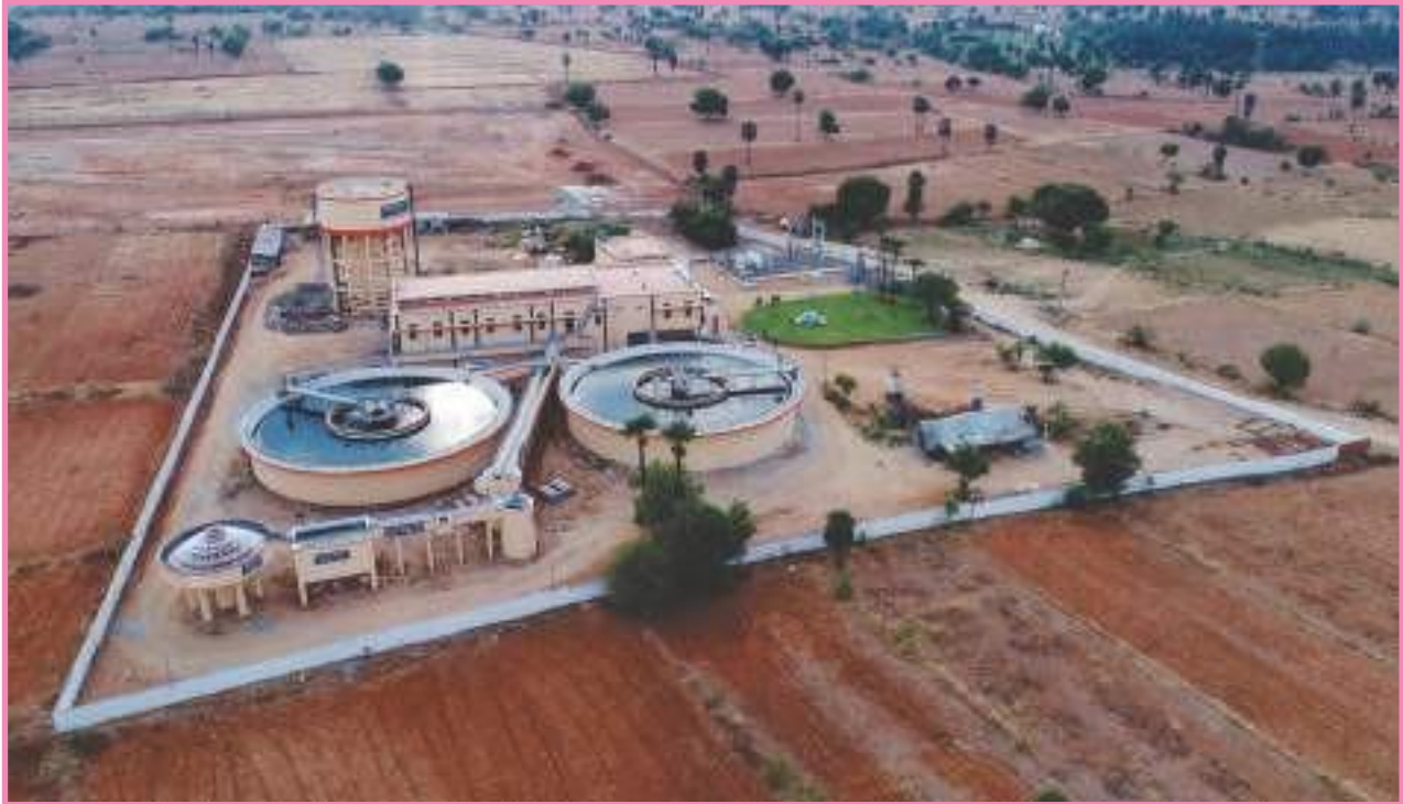
17.23 MLD capacity water treatment plant, constructed under CWSS to Perundurai and 7 other town panchayats including 547 rural habitations in Erode and Tiruppur districts.
